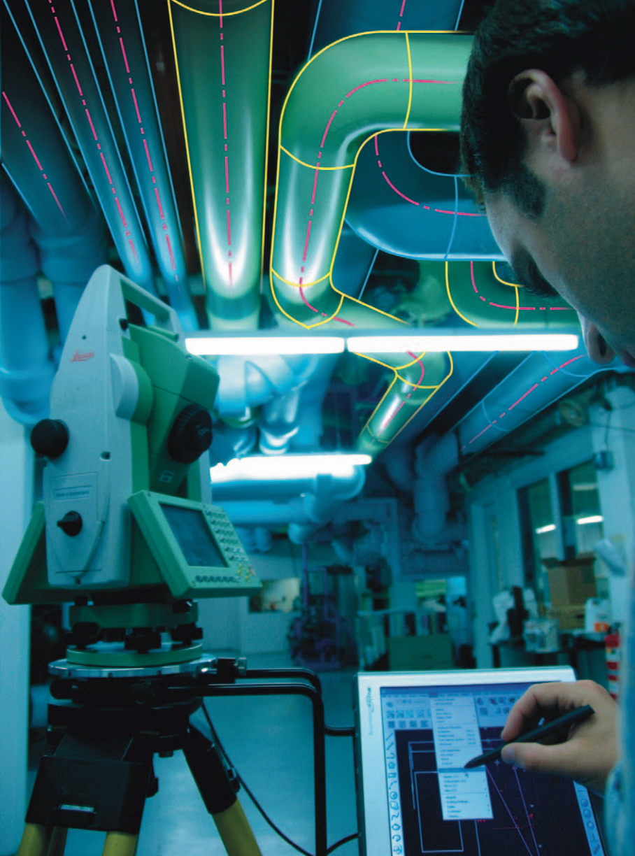
Figure 2. Reducing the steps between information capture and deliverables creation is key to effective as built creation.
